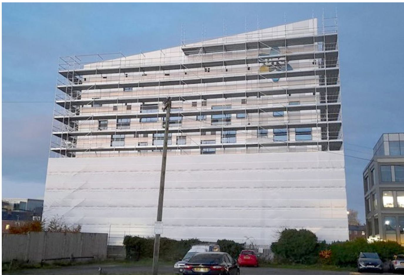
Photograph shows ITP's Powerclad Premium FR Scaffold Sheeting on an AT-PAC Ringlock system installed by Allied Access at a development by Conlon Construction
