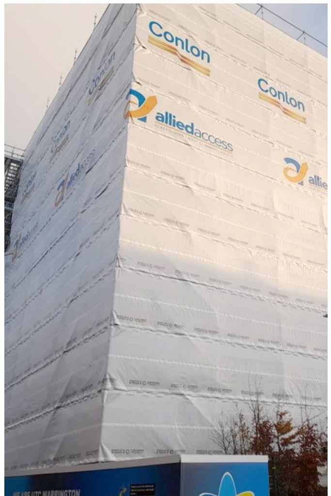
Photograph shows ITP's Powerclad Premium FR Scaffold Sheeting on an AT-PAC Ringlock system installed by Allied Access at a development by Conlon Construction
