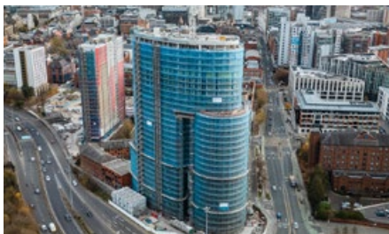
Crossway Scaffolding – Project Of The Year: Major
