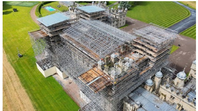
Infrastructure Site Services – Project of the Year: Major
