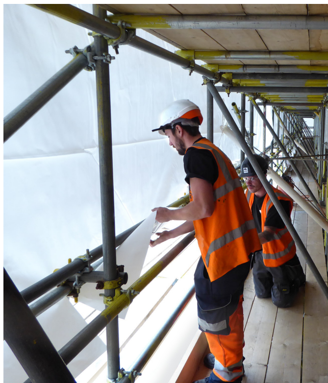
Figure 90: Showing good practice for fall protection during sheeting operations from a fully protected working platform. Source: Rhino
