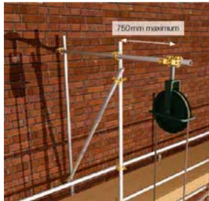
If a joint occurs in an inner standard between the horizontal gin wheel support and the lift below, the joint should be made with a sleeve coupler, rather than a joint pin, to resist uplift. Alternatively, a short section of tube may be spliced across the joint and connected with two swivel couplers or band-and-plate couplers.
