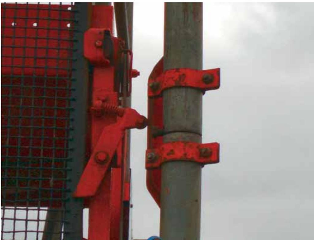
Figure 2 – Temporary Cage Gate Interlock Ramp for a Passenger Hoist Based TSTS
