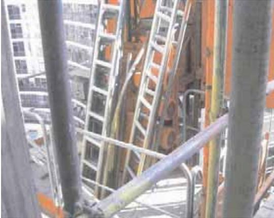
**Unsecured scaffold tube jammed in mast.**
