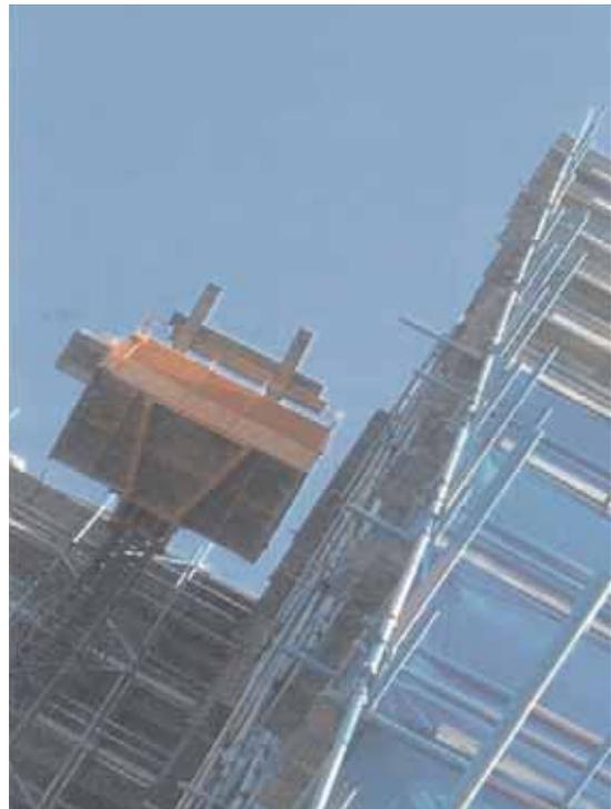
**Never allow materials to project outside the confines of the cage/platform. The overhanging materials may catch on a projection into the hoistway and fall onto people below.**
