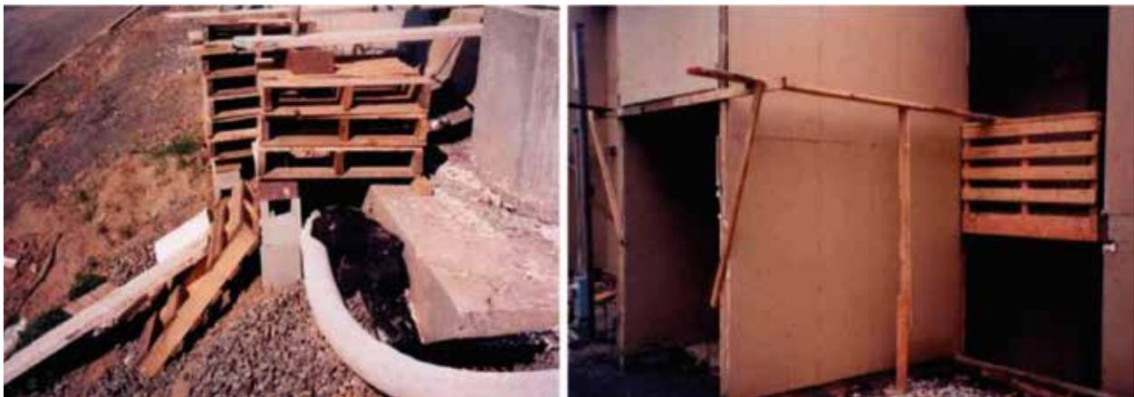
Figure 3 & 4. Loose material, insecure wooden frames, trailing cables etc.
