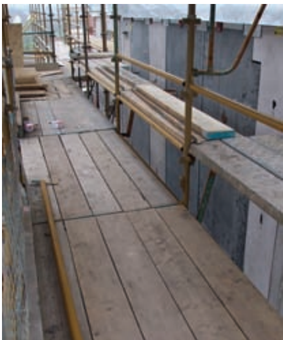
Removal of guardrails by other trades
