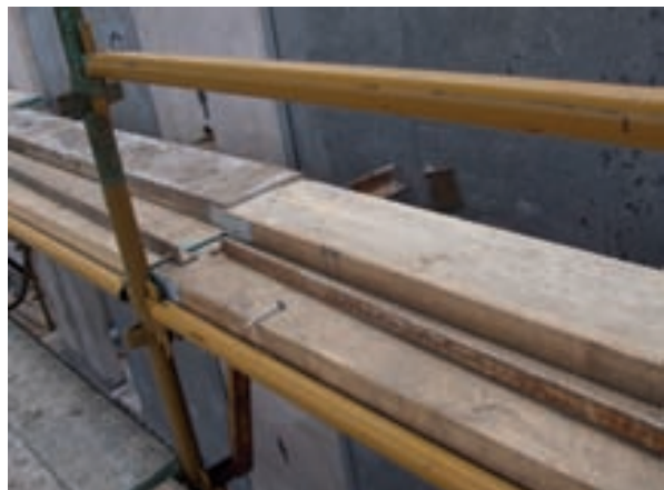
Removal of inside boards by other trades
