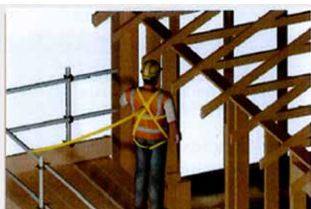
If an operative is required to work from an inner platform where the service gap exceeds 225 mm and presents the risk of injury, double guard rails should be provided at the inner platform edge connected with puncheons. Alternatively, a safe system of work must be employed that includes a full body harness and restraint lanyard to prevent the operative falling from the inside open edge, unless another suitable means of protection is determined from the risk assessment.
