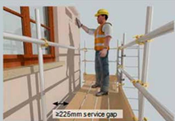
If the service gap exceeds 225 mm and presents a risk of injury, but not a risk of a person falling through the gap, a single guard rail may be required with a safe system of work that includes supervision, training and instruction.
