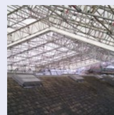
Scaffold Erection Services
