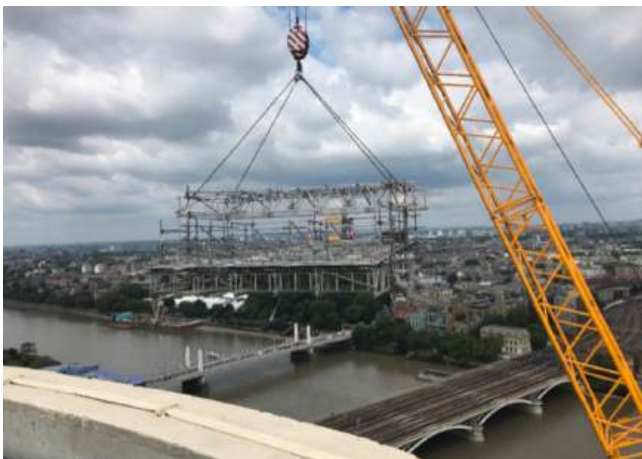
Figure 4: Example of pre-assembled modular sections of complex scaffolding lifted into place to avoid significant risks associated with working at height.
