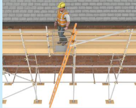
Example of a self-closing ladder safety gate.
